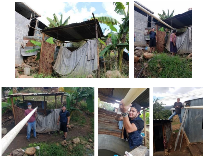
Figure 12. Improving Doña Mariana's rainwater collection system to supply water to her water tank and shower
